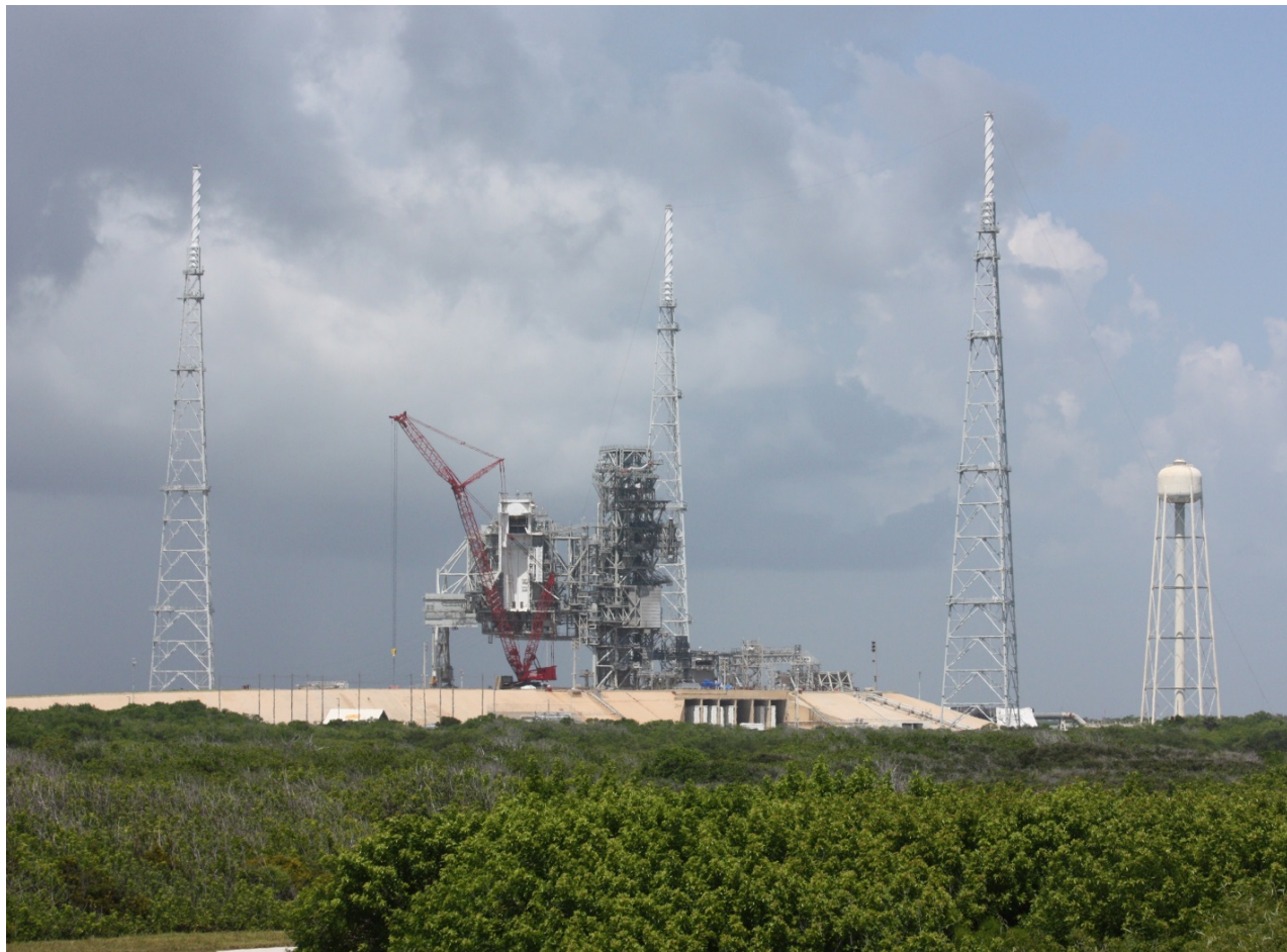
Lightning masts at Cape Canaveral Pad 39B. Image credit Wikimedia Commons ( source )
